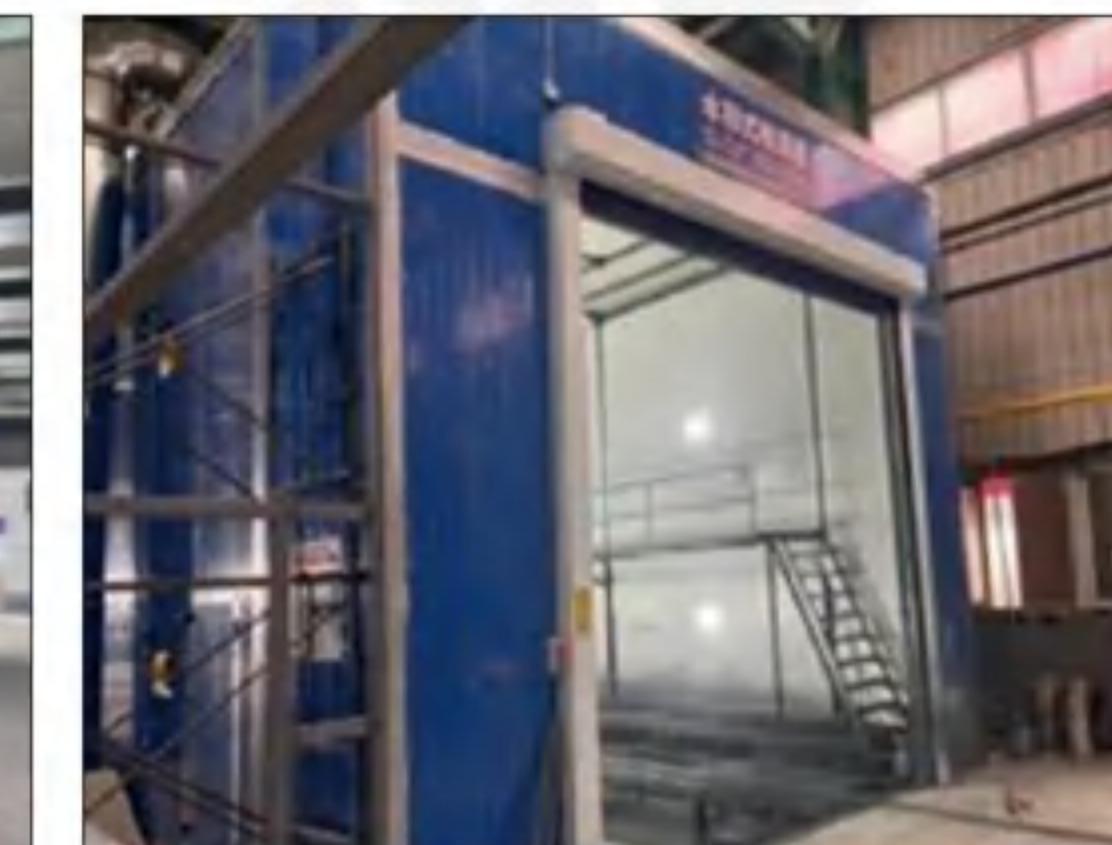
Painting station (18M) 喷漆站 (18M)
